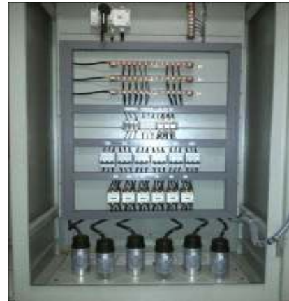
Gambar 4 a. Unit Kapasitor Bank Tipe Dynamic Var Compensator
